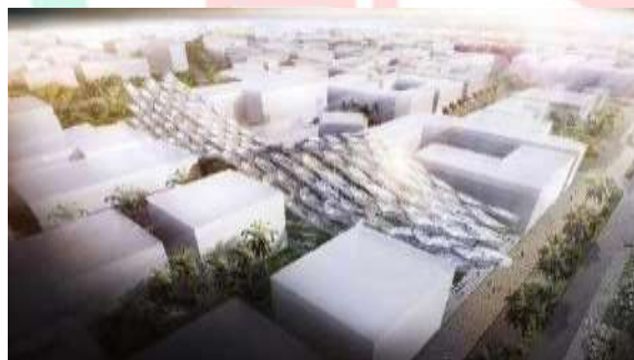
Gambar.2.2.3. 1 Fasad Surge Abu Dhabi (Sumber: archdaily.com, 2019)
