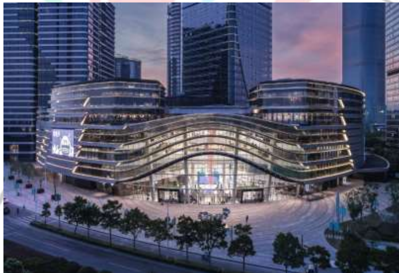
Gambar 2. 22 : Hong Leong City Center (Sumber : Archdaily, 2018)
