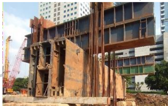
Gambar 3. 110 Posisi main beam, secondary beam, dan belimbing
