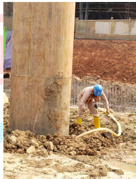
Gambar 3. 27 Cek kesentrisan casing
