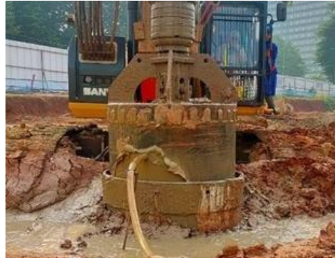
Gambar 3. 30 Penginjeksian polymer
