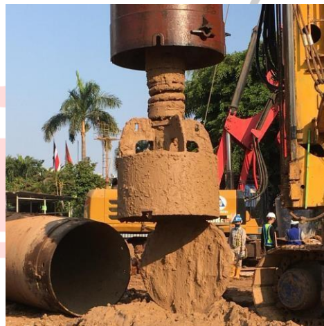
Gambar 3. 32 Proses pekerjaan cleaning
