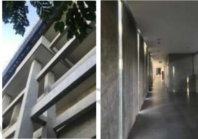
Gambar4.2 Beton dan Finishing Dinding
