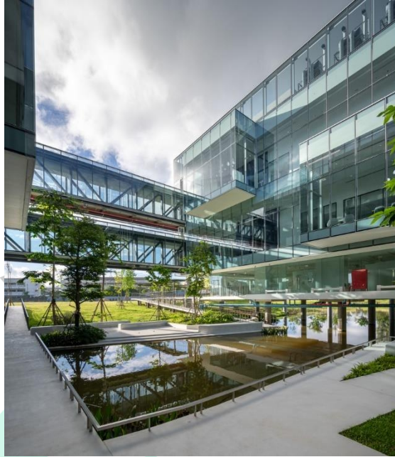
Gambar 2.15 Skybridge IRPC Innovation Center Sumber : (Archdaily, 2024)
