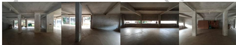
Gambar 3. 5 Area 1 Masjid Jami' Al-Hurriyah
