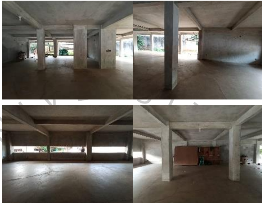
Gambar 4. 5 Area 1 Masjid Jami' Al-Hurriyah
