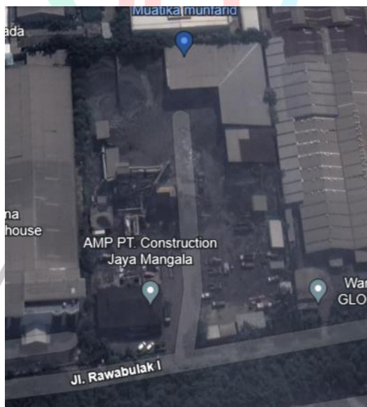
Gambar 3. 1 Laboratorium PT. Jaya Konstruksi Manggala Pratama Unit 1 Asphalt Mixing Plant
