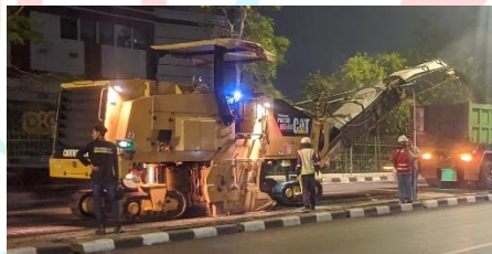
Gambar 3. 25 Cold Milling Machine (Source: Dokumen Pribadi)
