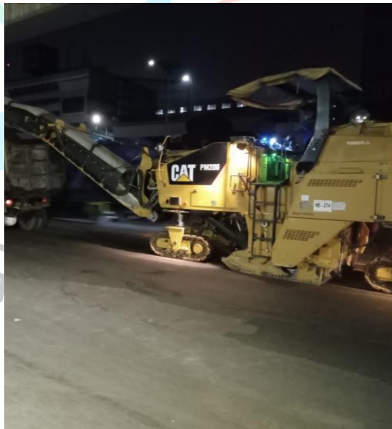
Gambar 3. 10 Cold Milling Machine (Sumber: Dokumen Proyek Jalan Rasuna Said, 2023)
